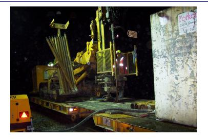
Site investigation drilling to investigate the presence and condition of coal workings under the Mostyn rail line in North Wales.
